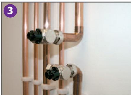
**3** Prepare the pipe and fittings accordingly. Lubricate the olives and assemble the valves on the pipe. Hand tighten.
